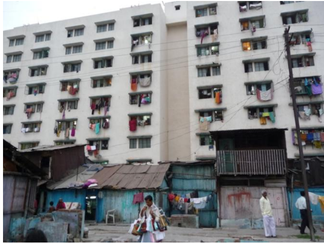
Figure 3: High rise in-situ rehabilitation buildings at Nanapeth, Pune, India.
